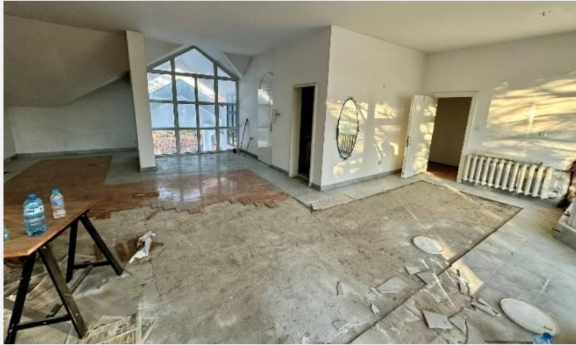
BRC's Community Centre before renovation. Source: BRC
